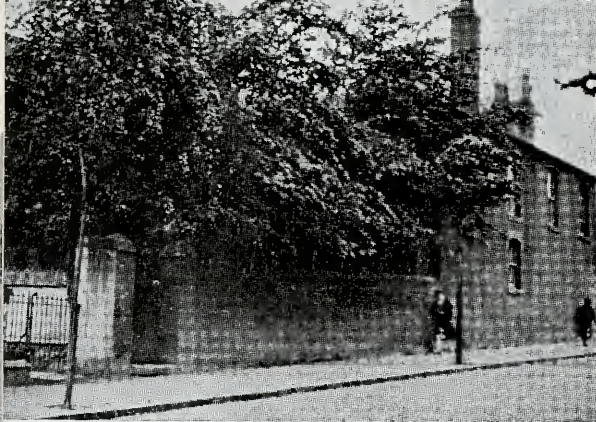
No. 23 Booth Street, Handsworth, Birmingham British Mission Headquarters from 1929 to 1932
